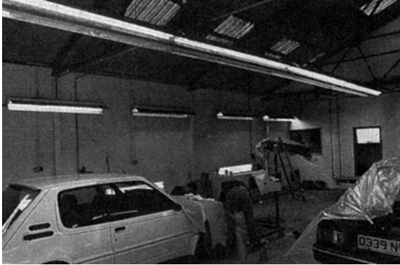
Figure 15.3 Lighting used in the stripping and straightening areas ( Fifth Generation Technology Ltd )
