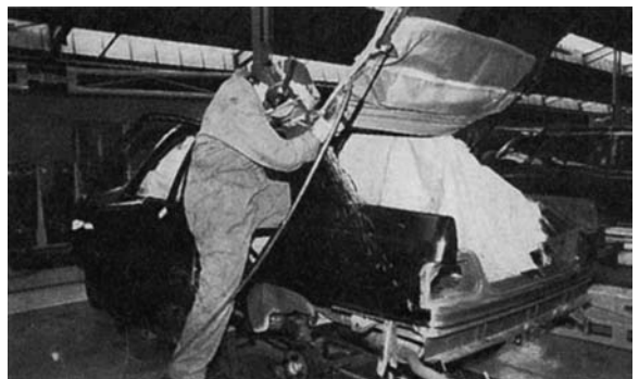
Figure 14.99 Cleaning up the locating flanges ( Motor Insurance Repair Research Centre )
